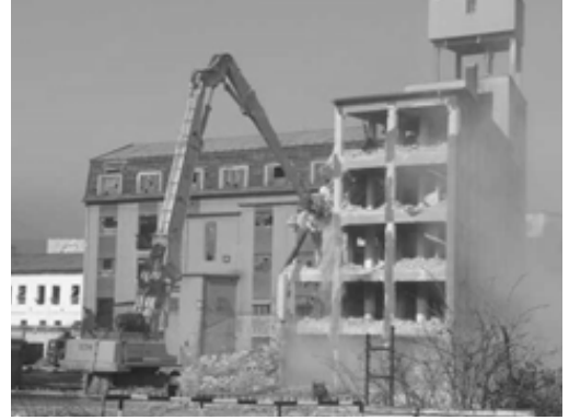
Figure 2. Demolition of the bakery Jedľa
