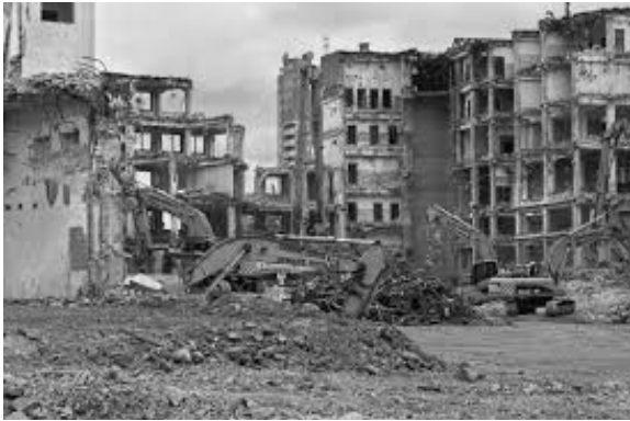
Figure 1. Demolition of the Stein Brewery
